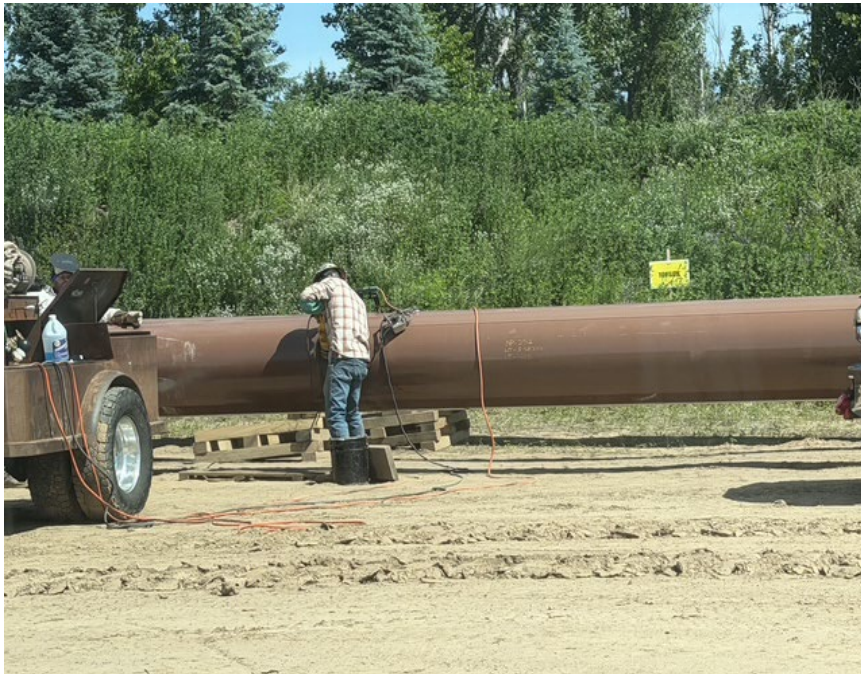
Facing north near MP 3.12, welding continues
