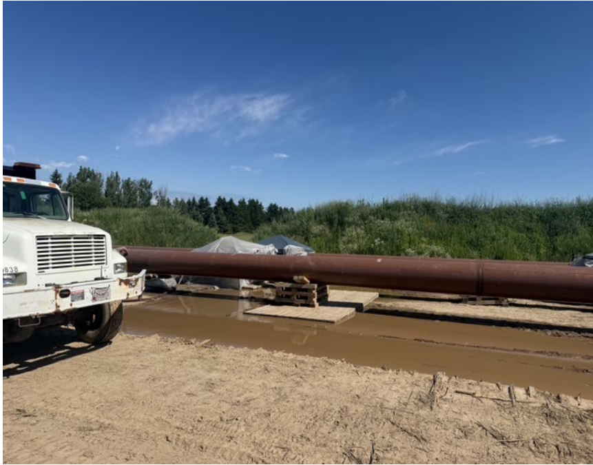
Facing north near MP 3.12, sandblasting commenced
